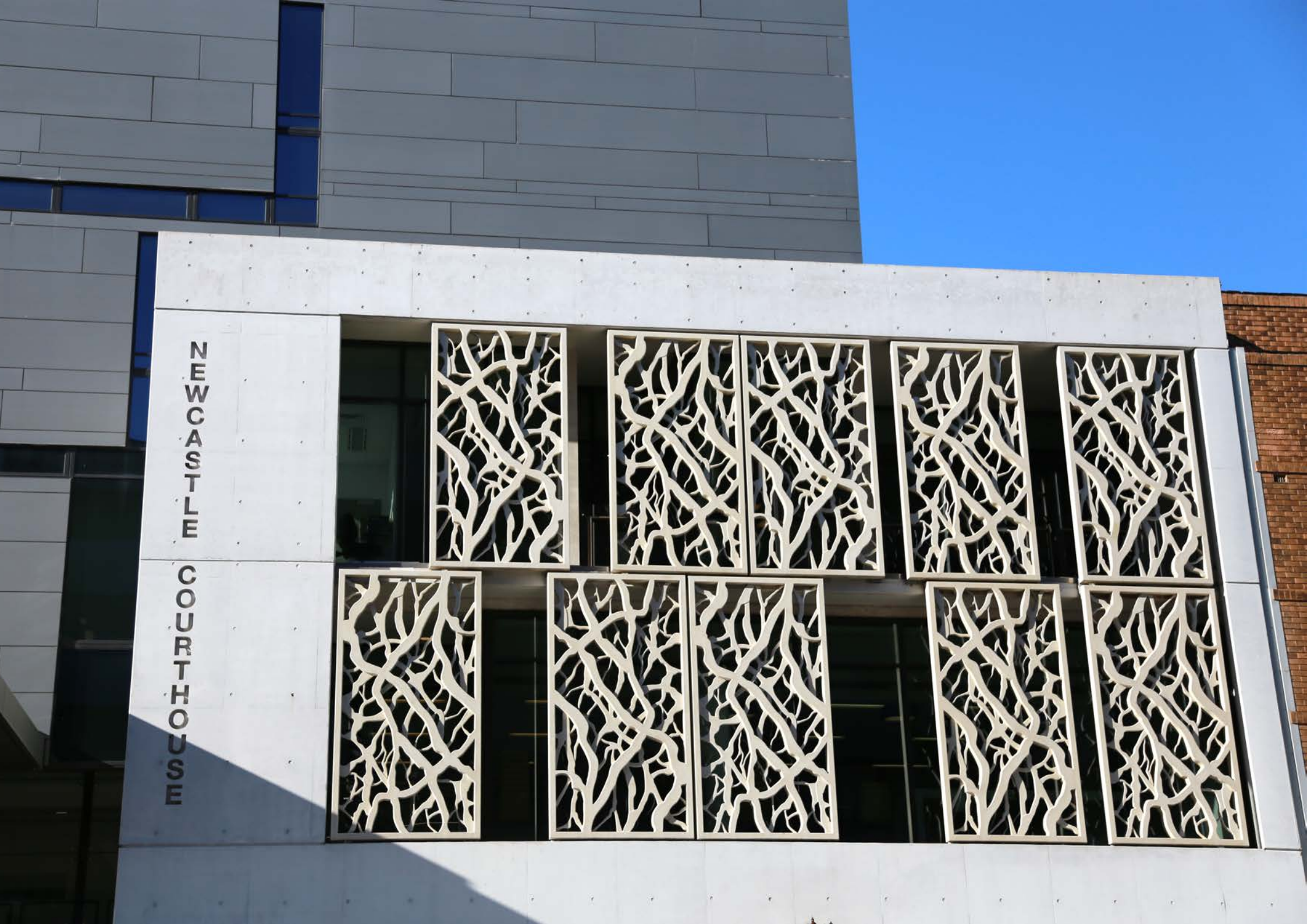
Newcastle Courthouse facade from Hunter Street. Credit: Claire Albrecht
