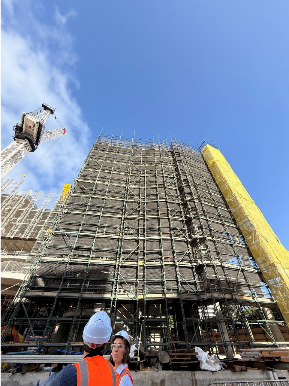
Photograph B.2 Building works
