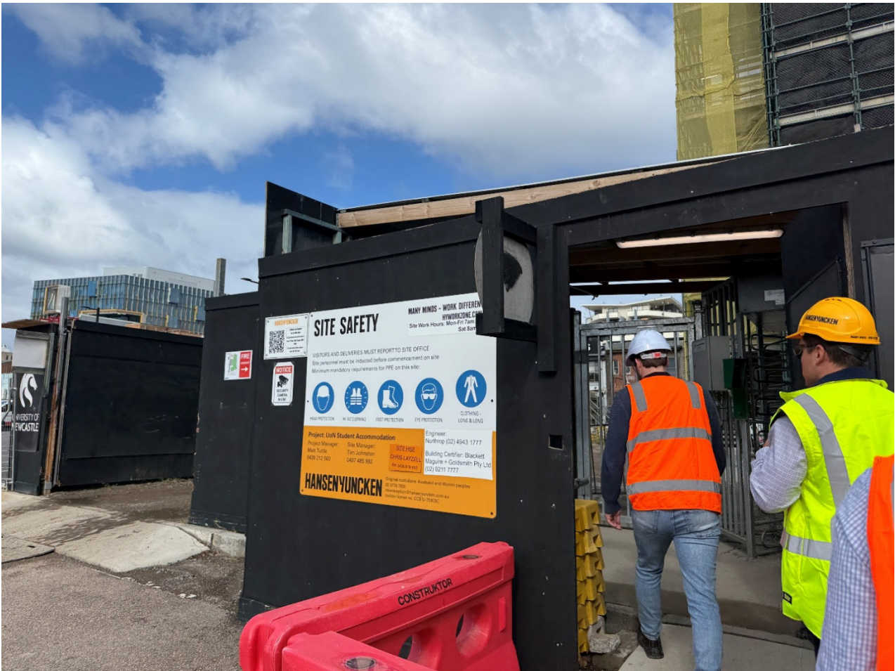
Photograph B.3 Entry to construction zone (gate open)
