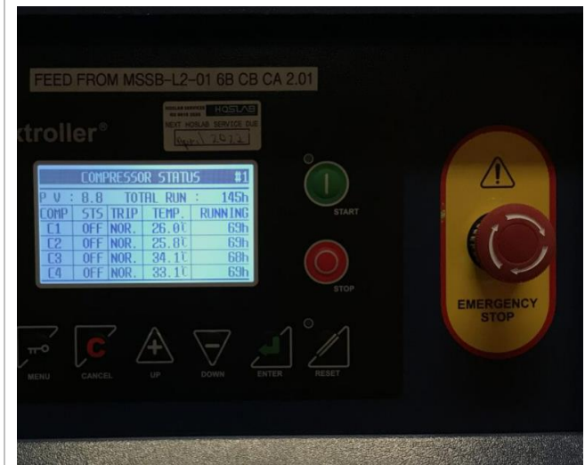
MSSB-L2-01 compressor status as normal
