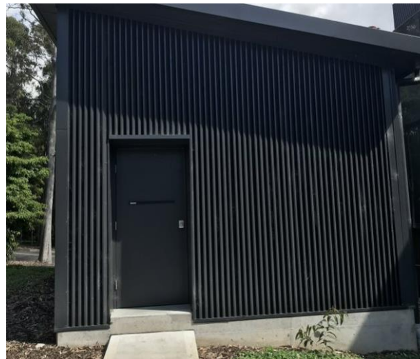
Generator stored securely in standalone shed.
