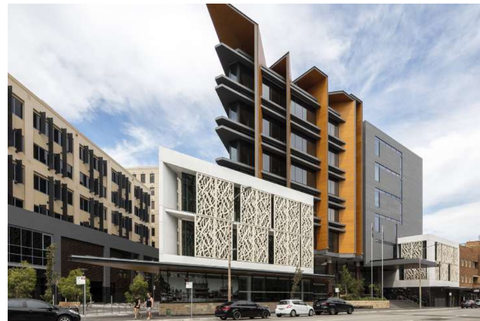
Neutral materials palette with differentiation between podium and upper levels Newcastle Courthouse
