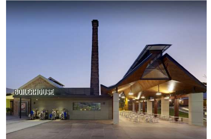
Boilerhouse heritage adaptation, WSU Rydalmere
