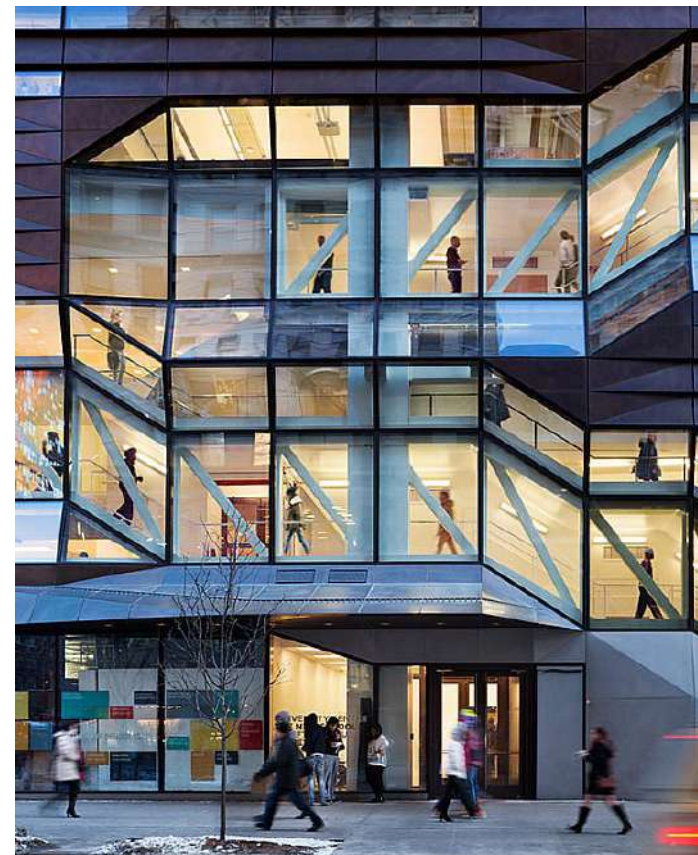
Facade transparency shows internal vertical circulation. The New School University Centre, NY
