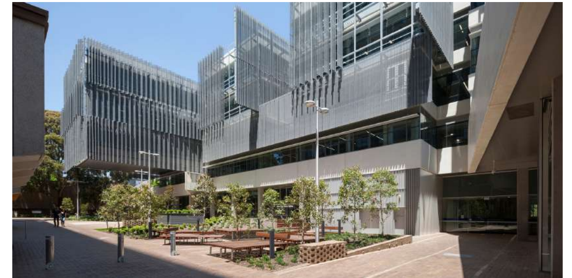
Building screening creates comfortable internal spaces, while ground level planting enhances biodiversity and regulates the microclimate. Melbourne School of Design, University of Melbourne
