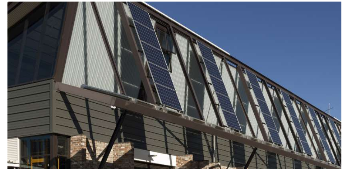
Photovoltaic cells are integrated with the roof form to enable energy collection Sustainable Buildings Research Centre, University of Wollongong, photographer: Richard Glover
