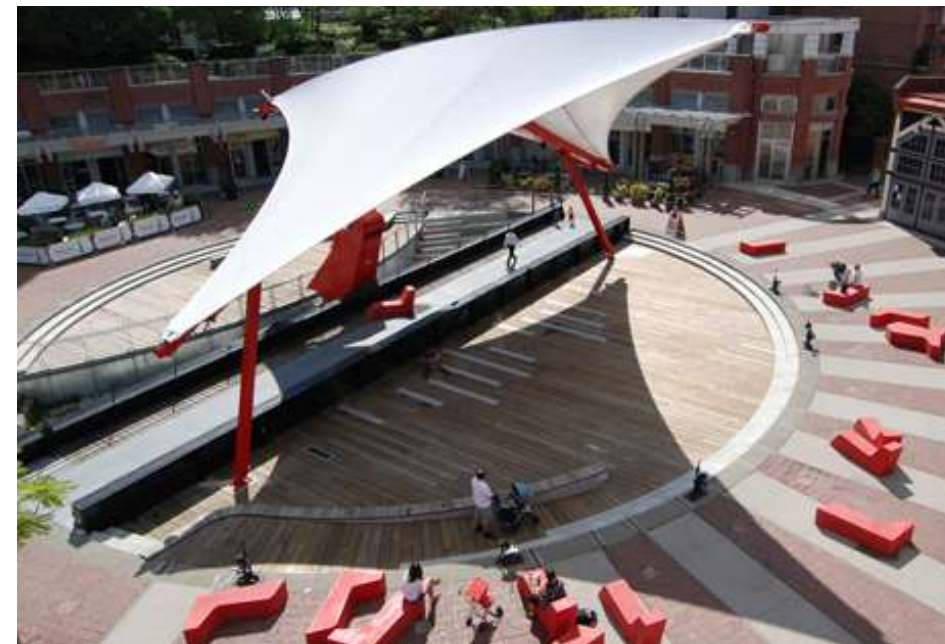
Heritage interpretation of former turntable, Roundhouse Turntable Plaza Vancouver
