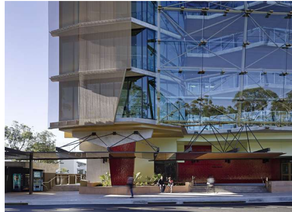
Glazing with sun shading screening provided to exposed facades Sir Samuel Griffith Centre
