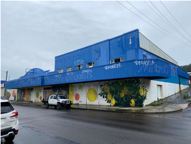
Picture 1 View of the site from the corner of Mann and Hills Street
