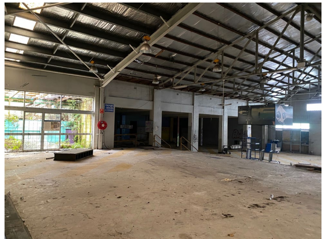
Picture 4 Within the existing building on the site
