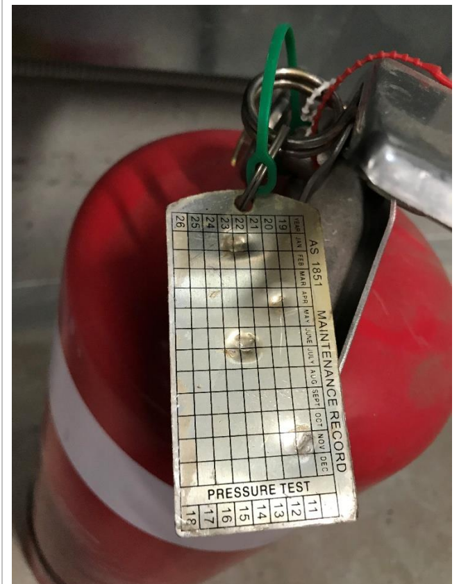
Fire extinguisher tag current (last checked June 2022)
