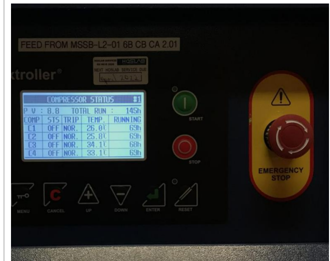
MSSB-L2-01 compressor status as normal
