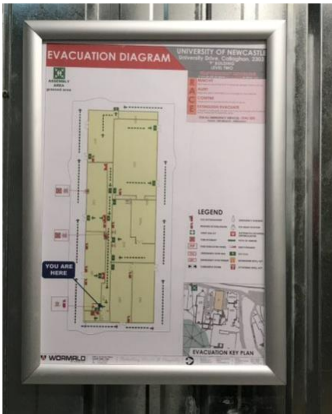
Evacuation plans located in every plant room
