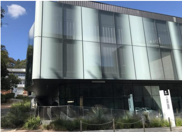
Façade of Bioresource Facility (F Building)
