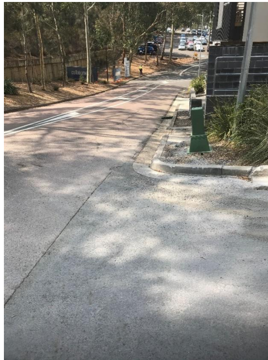
Photo 5 - Sediment controls provided in stormwater drains
