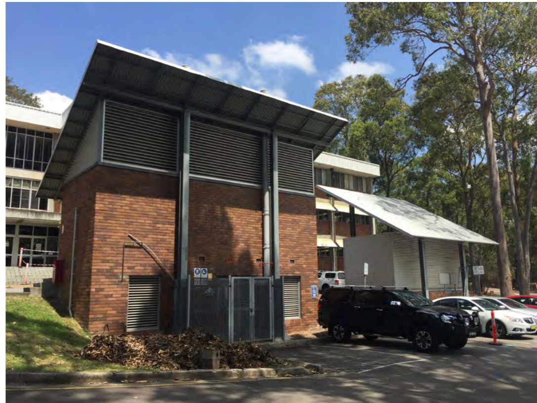
08_View from the south car park to the south west showing existing service buildings
