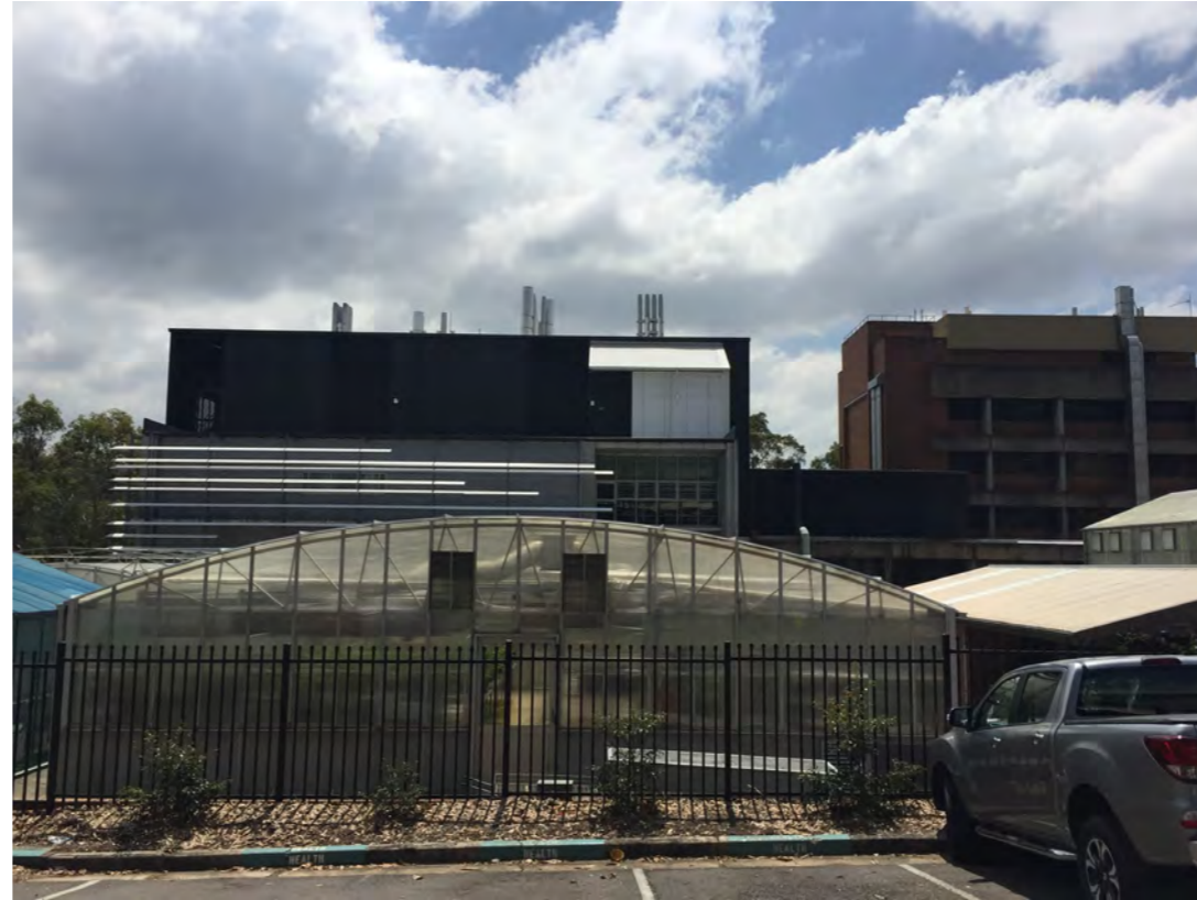
06_View from the south car park to the north towards the Medical Sciences West building
