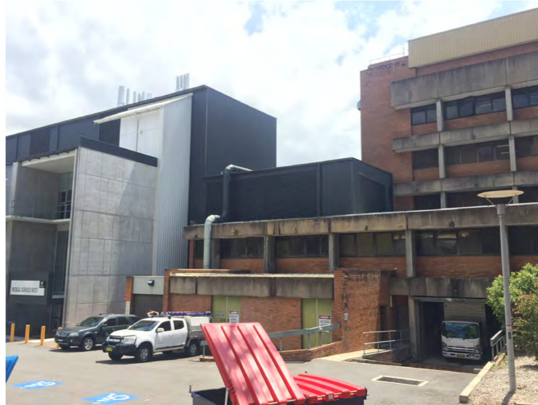
14_View from Medical Sciences Lane (Service Road) towards the Medical Sciences loading dock
