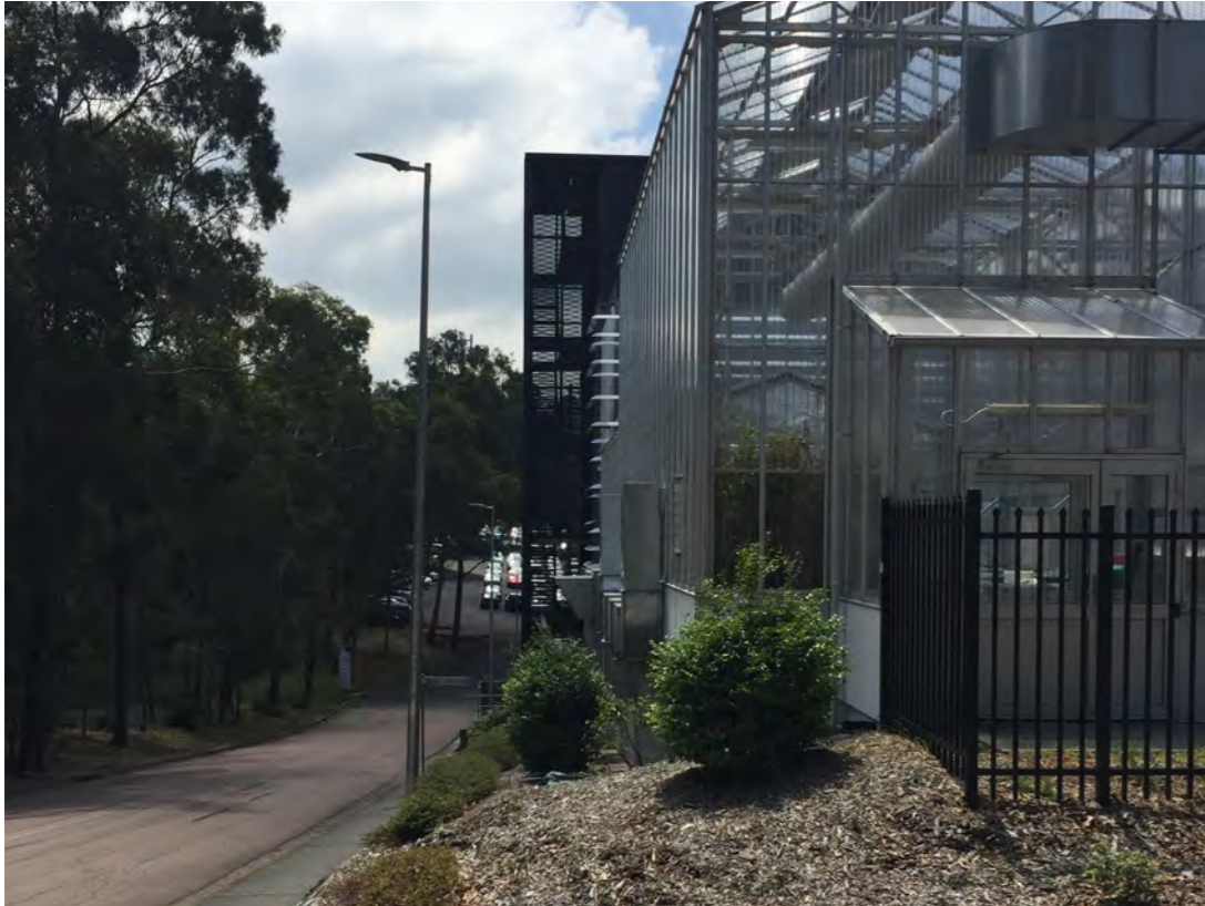
05_View from the car park access road to the north showing existing building alignment
