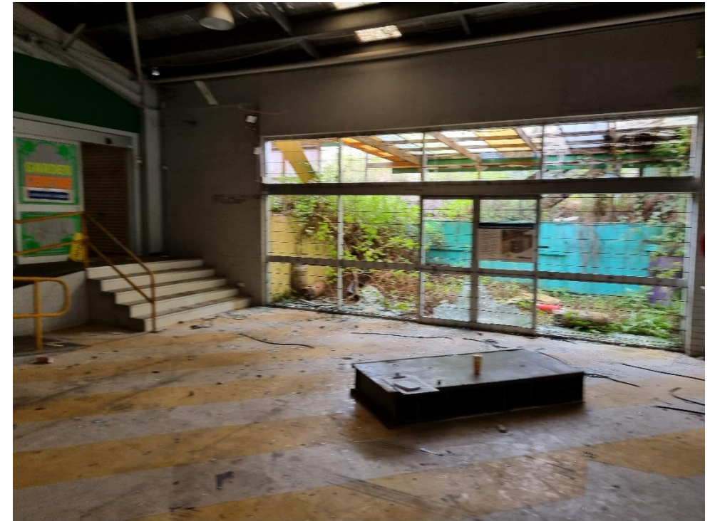
Photo 9: Former southern patio of Site. This portion of Site is heavily disturbed with overgrown vegetation and smashed glass.
