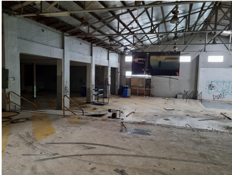
Photo 8: Southwestern portion of the Site's main structure. Main entrance is visible in this image and has been bordered to restrict access.
