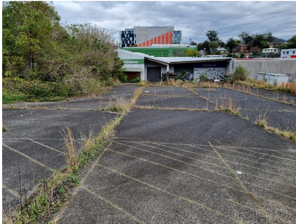
Photo 2: Northeast corner of Site facing the main structure to the west.
