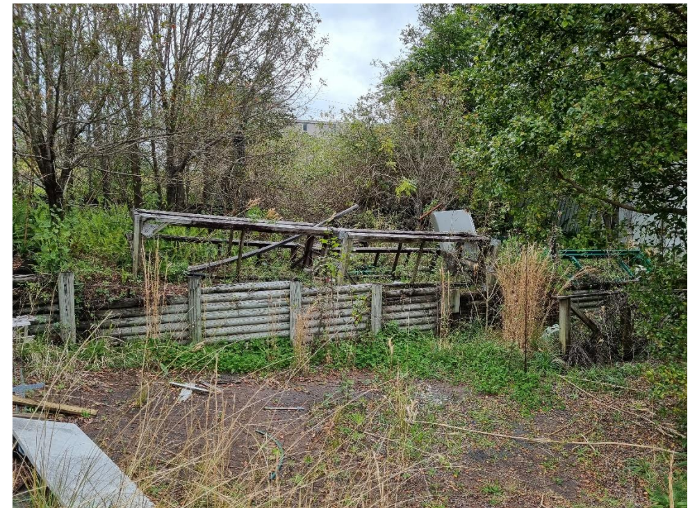
Photo 6: Historical retaining wall inside central vegetated area of Site.
