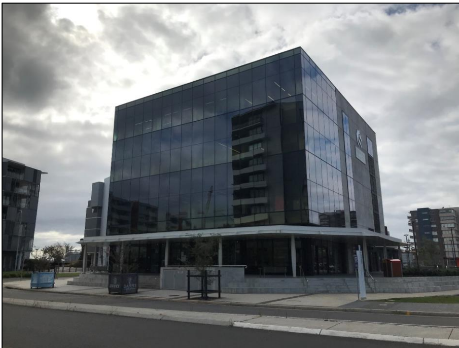
Figure 4 – General external photo of building (west)
