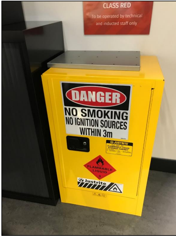
Figure 9 – Hazardous materials storage cabinet (Maker Space)
