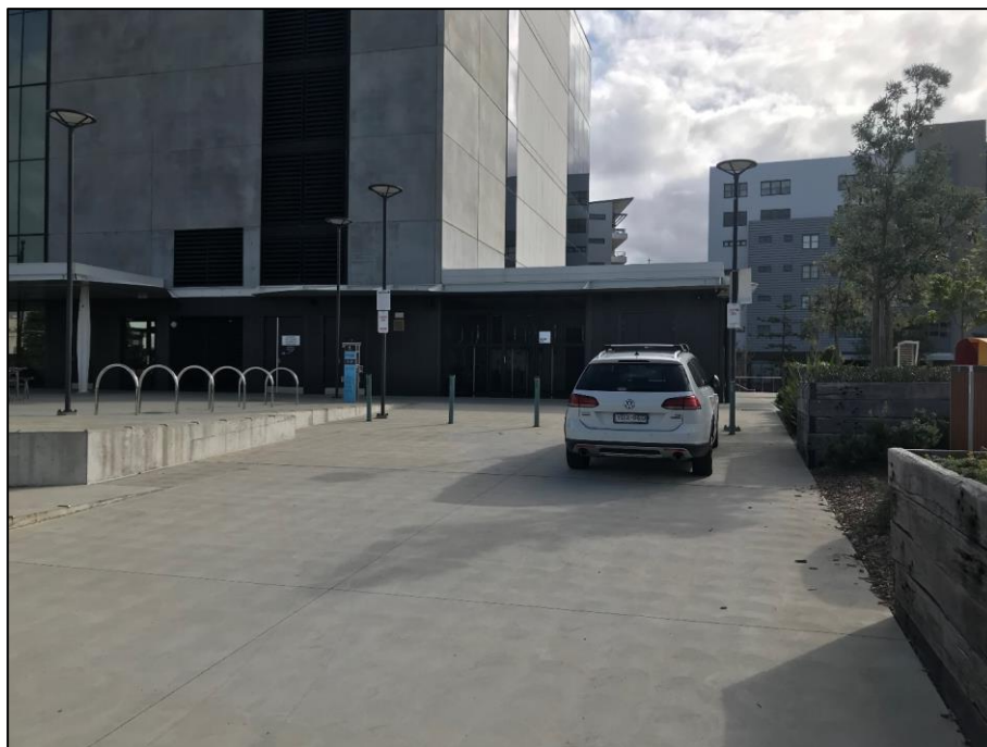
Figure 19 – Southern loading zone
