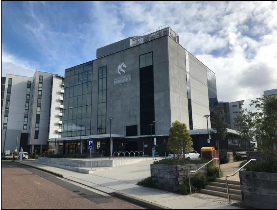
Figure 3 – General external photo of building (south)
