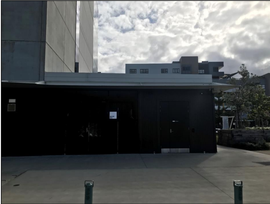
Figure 11 – Bin store (external)
