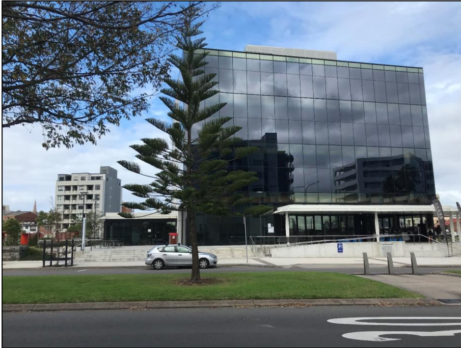
Figure 5 – General external photo of building (north)
