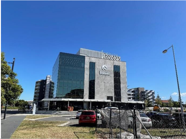
Building façade viewed from South.
