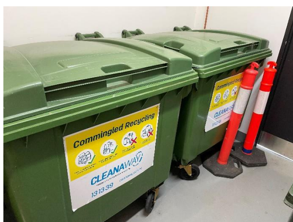
Commingled recycling bins in waste storage room
