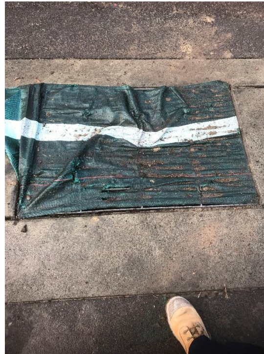
Photo 5 - Drains were covered to prevent sediment entering
