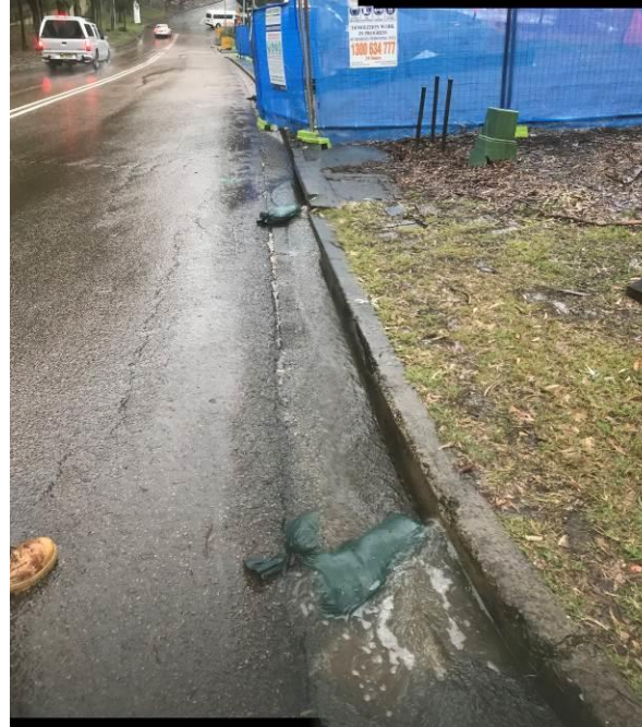
Photo 8 – Sediment controls provided in stormwater drains
