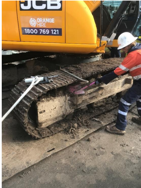
Photo 1 – Cleaning excavator prior to removal from site
