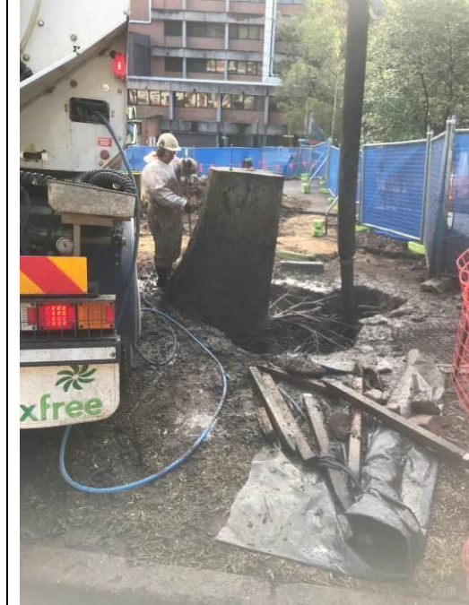
Photo 9 – Tree stumps and roots removed by hydrovac.
