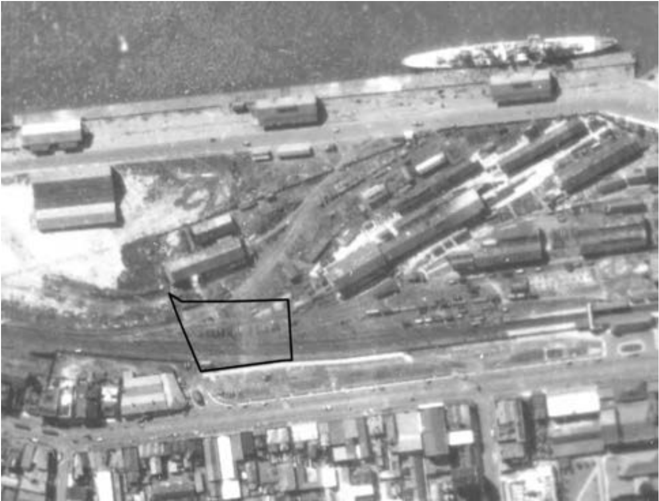
Figure 2.3 Detail of 1938 Aerial Photograph
