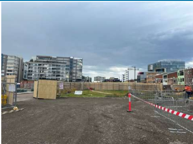
2025 (current) photograph to east showing protected fenced area (exclusion zone) within the Project Area Umwelt 2025
