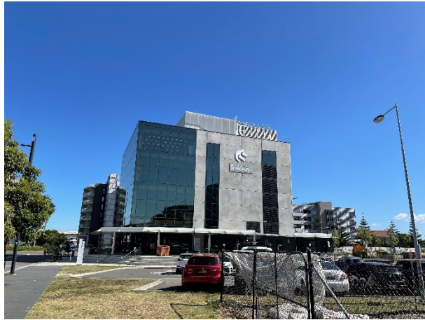
Building façade viewed from South.
