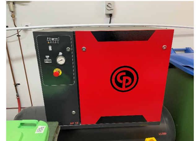
Cardboard compactor in waste storage room.
