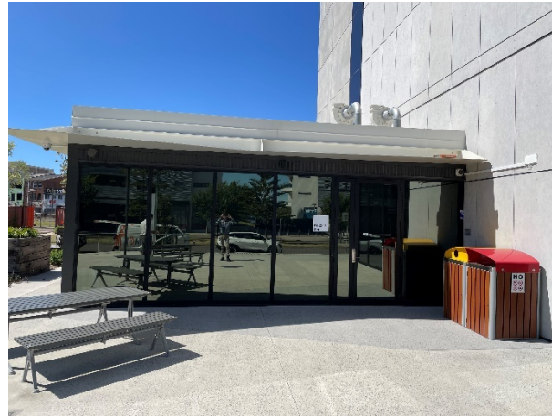
Temporary building extension for maker space and bike shed.
