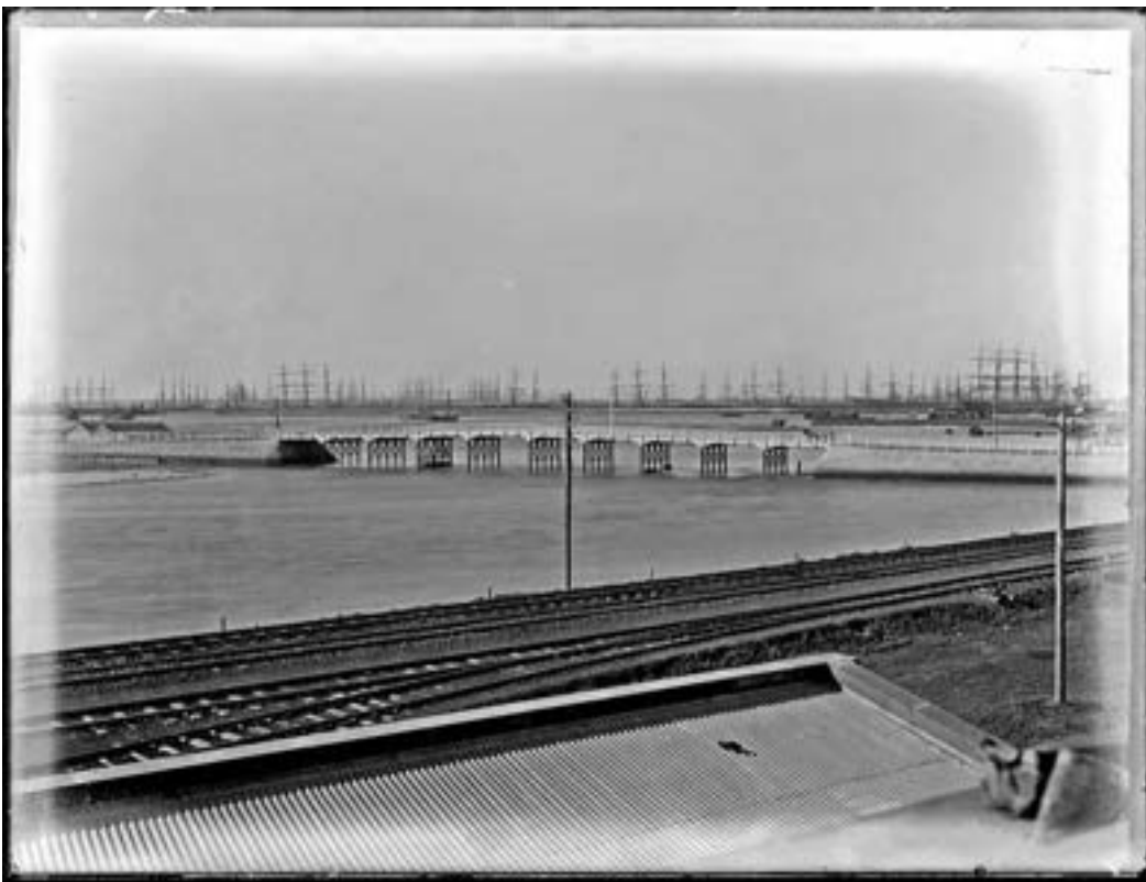
Figure 3.10 View of the new Bullock Island bridge across Throsby Creek in 1900 The new bridge was timber on iron piers.
