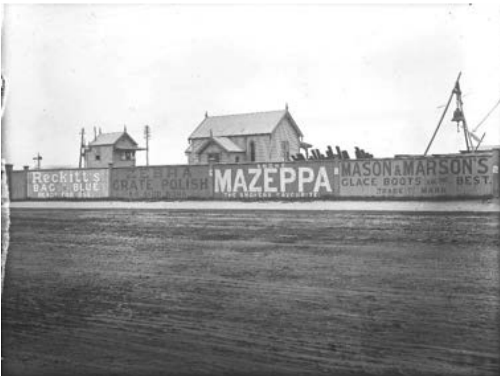
Figure 3.13 1896 Photograph showing Mortuary Station
