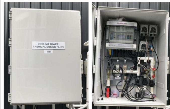
Cooling tower chemical dosing panel secured and suitably accessible for maintenance
