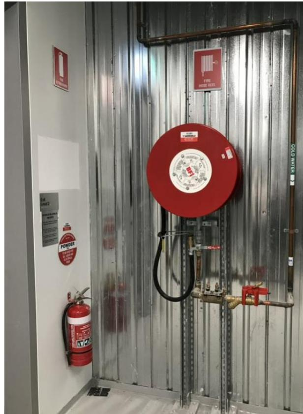
Accessible fire extinguisher and fire hose in plant room
