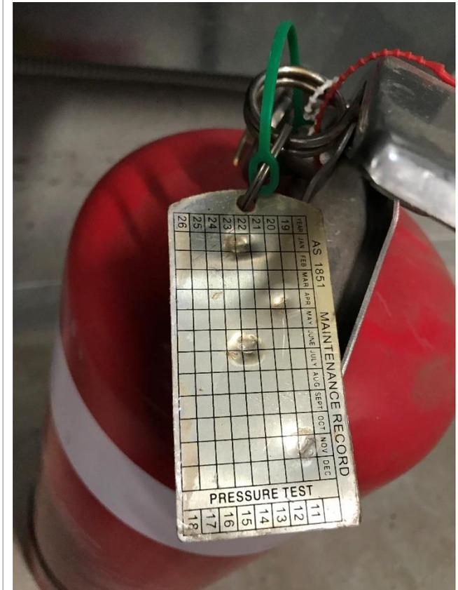
Fire extinguisher tag current (last checked June 2022)
