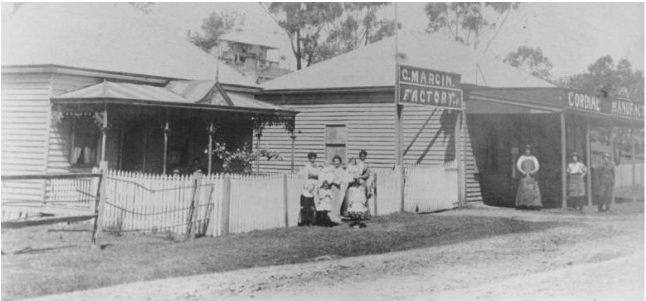
Figure 18 – Historic image of the subject site in 1906, showing the Margins' Cordial Factory and Ice Works. This image shows the cottages which front Hill Street, and remained present at the site until the late 1990s.
