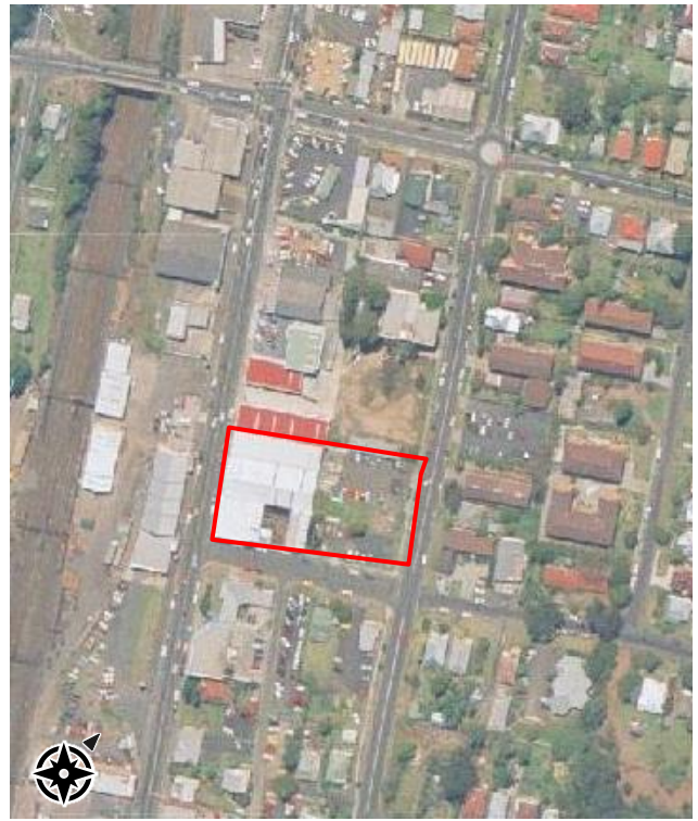
Figure 29 – Historical aerial of Gosford from 1994, showing the subject site including a large carpark spanning Lots 30-32.
