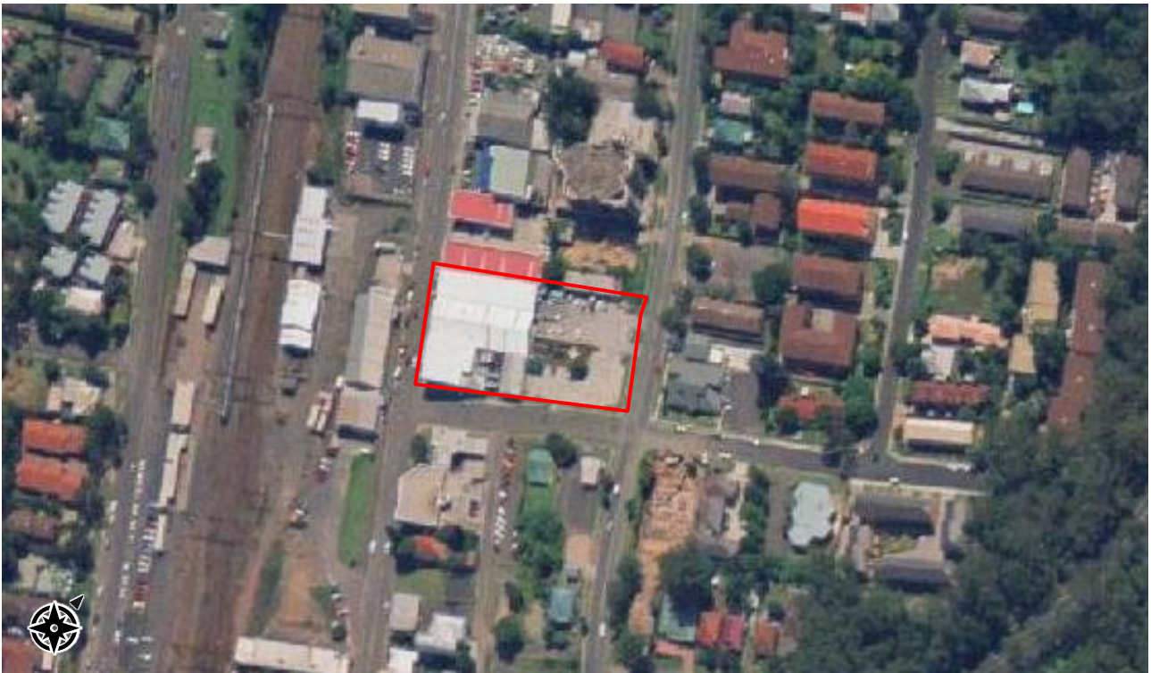
Figure 30 – Historical aerial of Gosford from 2002, showing the subject site including a large carpark spanning Lots 30-32.
