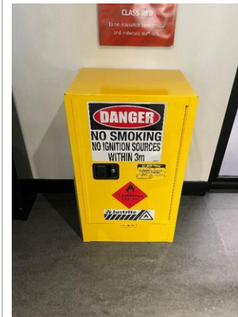
Hazchem cabinet in 3D printer workspace.
