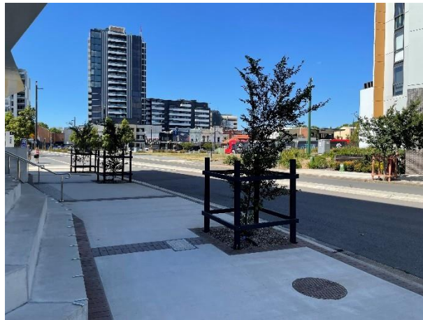
Street trees (landscaping) and protection in good condition.
