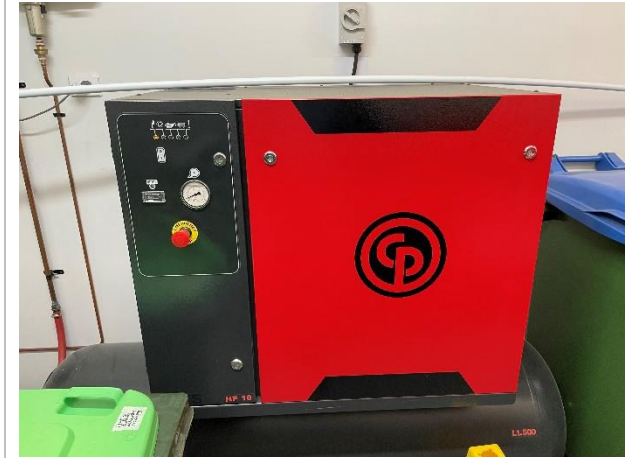
Cardboard compactor in waste storage room.
