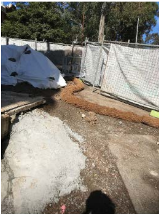
Evidence of Sediment Controls in place
