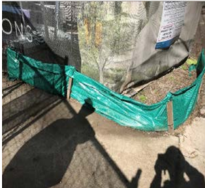
Evidence of Erosion and Sediment Controls
