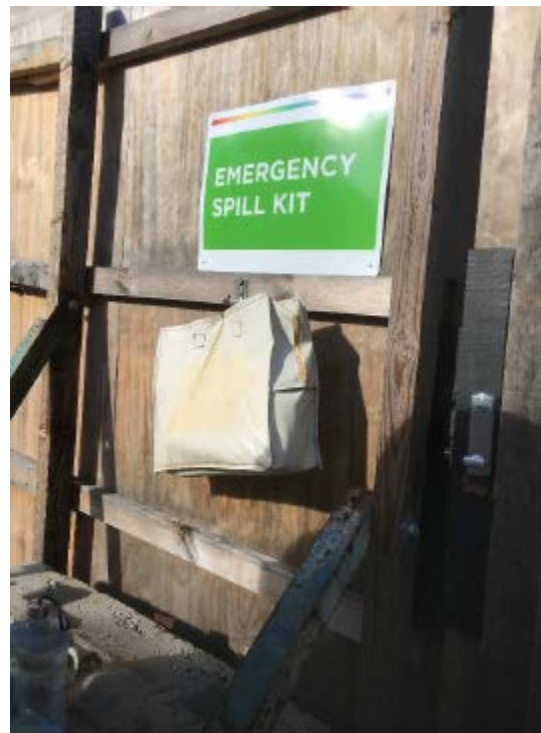
Evidence of Spill Kits on site
