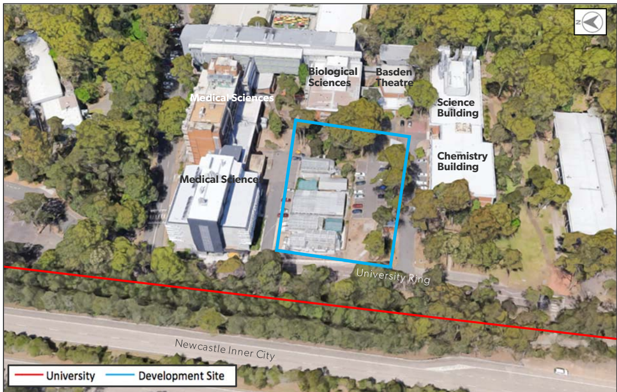
Figure 4 | Aerial view of site from the west (Base source: Google Maps)
