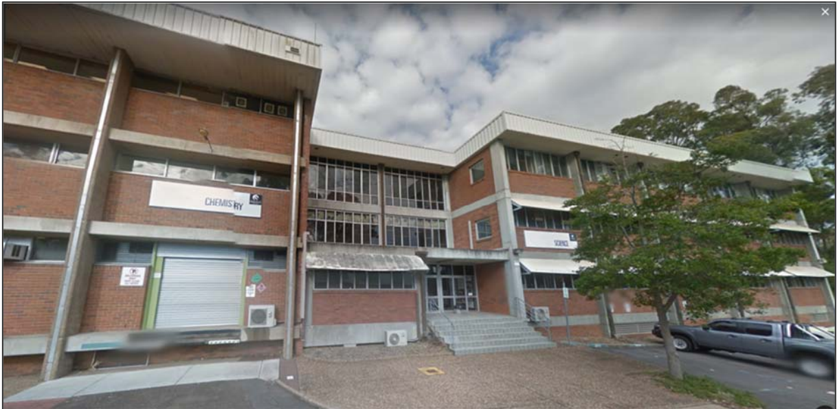
Figure 10 | Chemistry and Science Buildings (Source: Google Maps/streetview)
