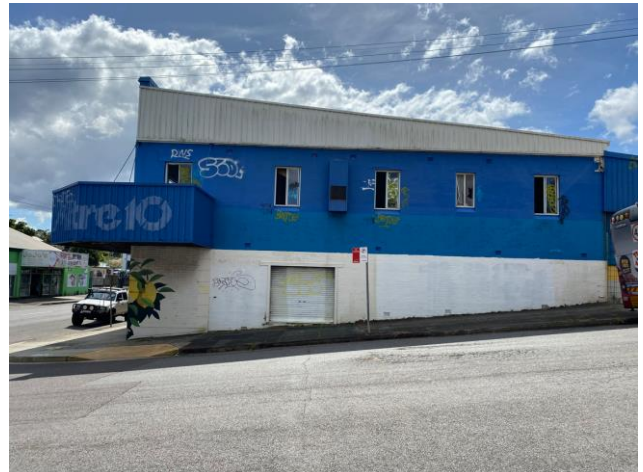
Figure 17 View north showing Beane Street elevation.
