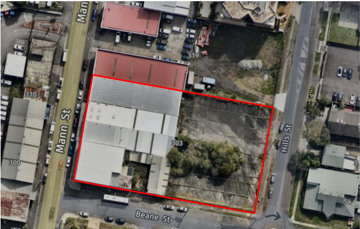
Figure 13 Aerial imagery of subject site.
