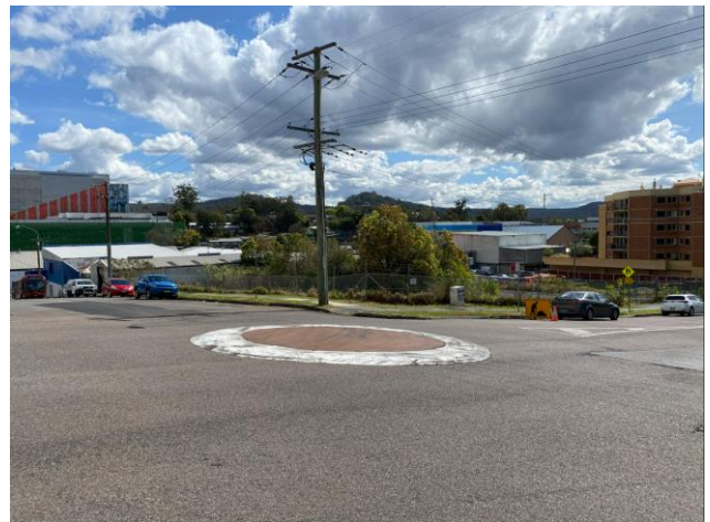
Figure 10 View north-east towards subject site from corner Beane and Watt Street.
