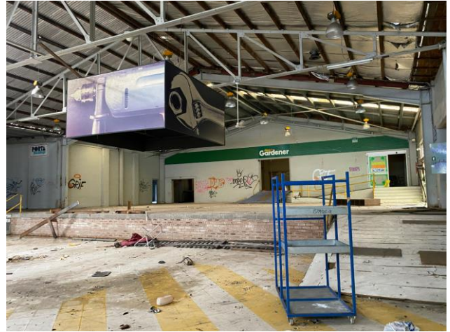
Figure 26 View towards area B2 from B1.
