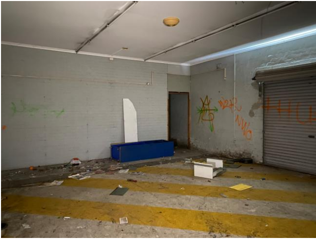
Figure 27 Interior spaces, south-eastern quadrant of site.
