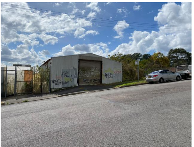
Figure 20 Shed along southern boundary.
