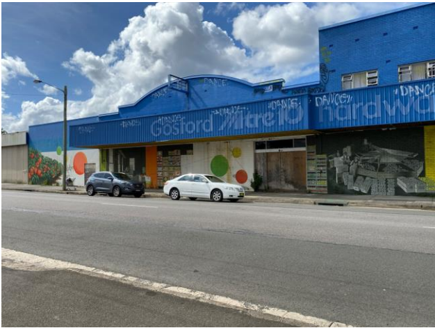
Figure 16 View north-east showing arched parapet at Mann Street elevation.
