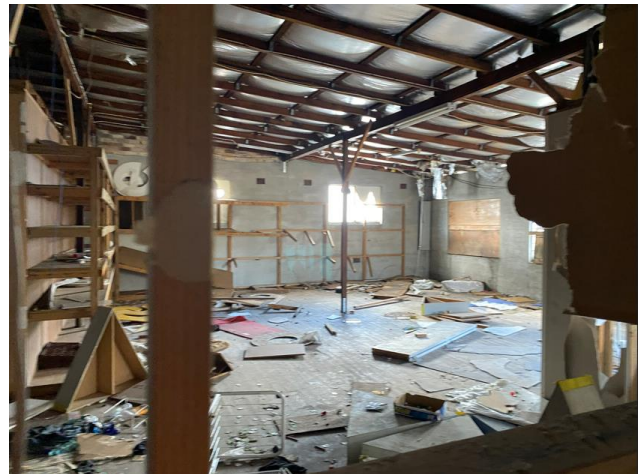
Figure 36 First floor interior fabric, view north-west.
