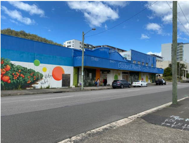
Figure 14 View south-east along Mann Street.
