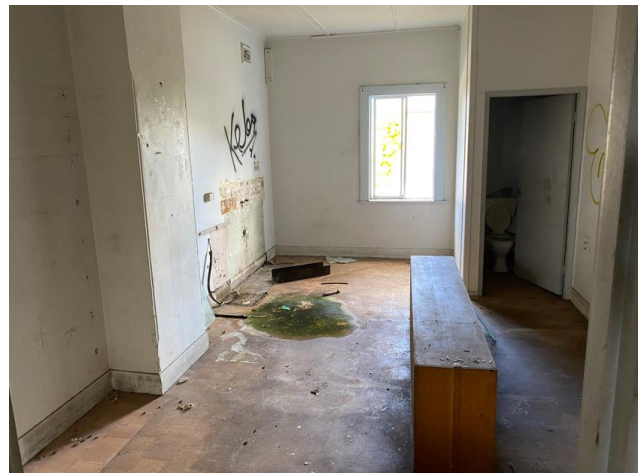
Figure 38 First floor interior rooms.
