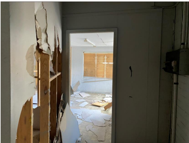
Figure 37 First floor interior rooms.
