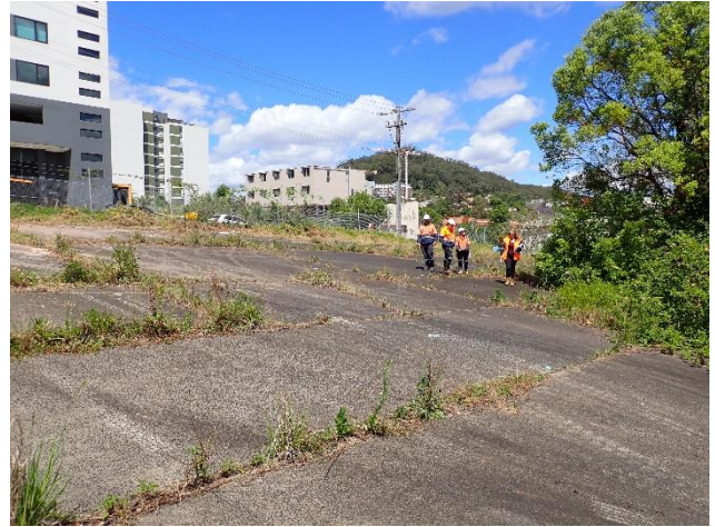
Figure 19 – Hardstand conforms to landscape topography.
