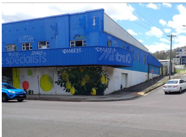
Figure 16 – Variation in levels indicating ground disturbance. View north east.
