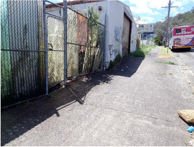
Figure 18 – Cut and fill levelling. Southern boundary.
