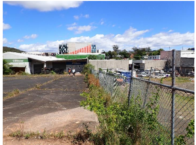
Figure 21 – Adjacent property cut down to create a level surface.
