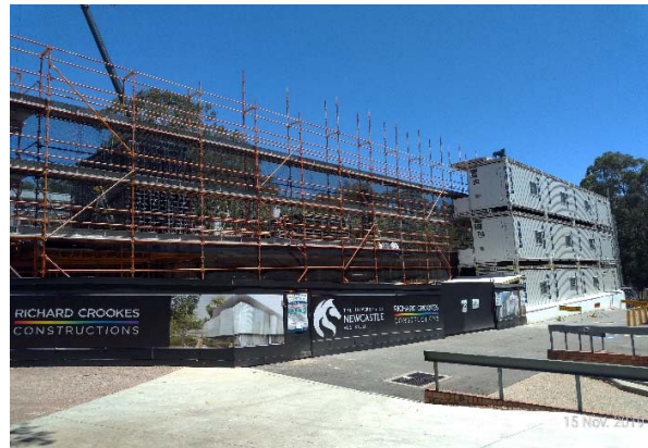
C13 – Evidence of Construction Hoarding
