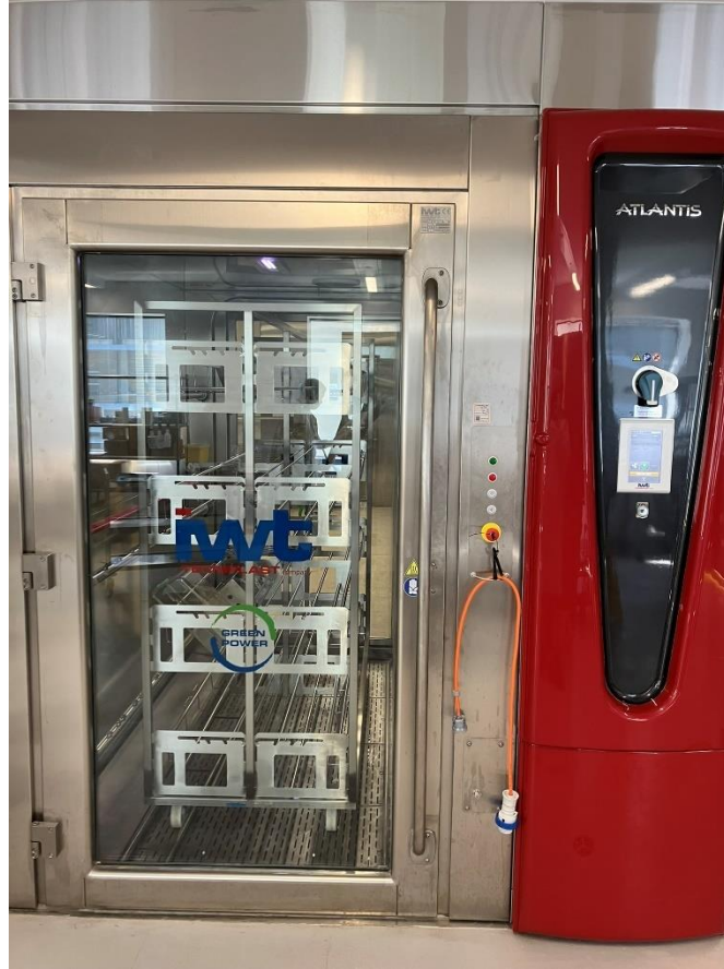
Figure 38 Steriliser in PC2 Zone
