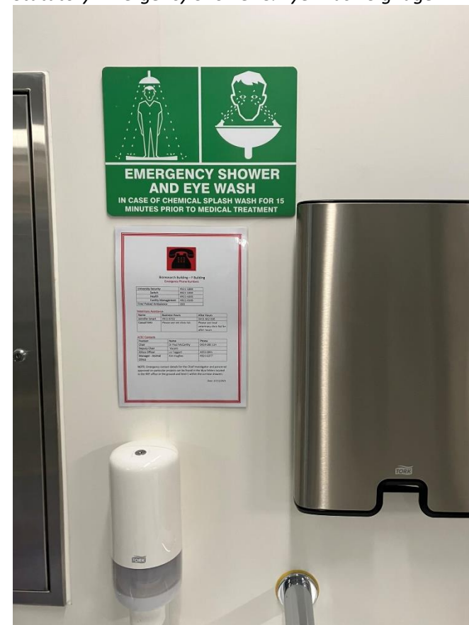
Figure 24 Statutory Emergency Shower & Eye Wash Signage
