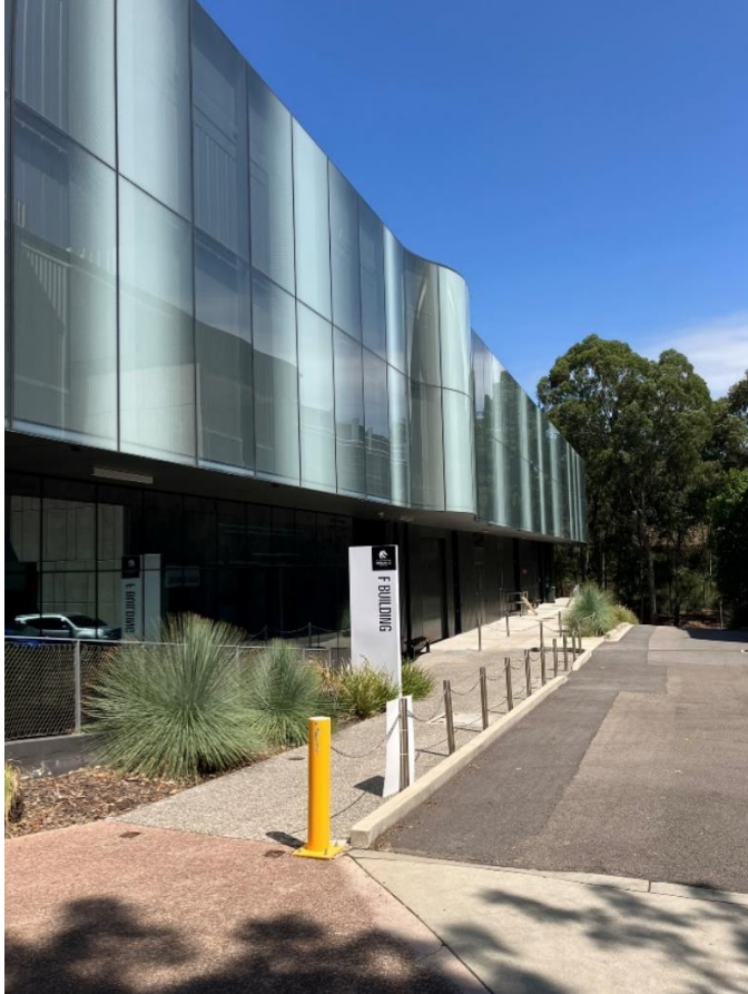
Figure 4 External perimeter kept clear and clean
