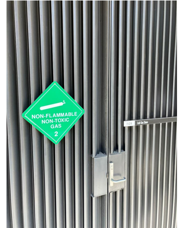
Figure 18 External Signage – Non-flammable Gas
