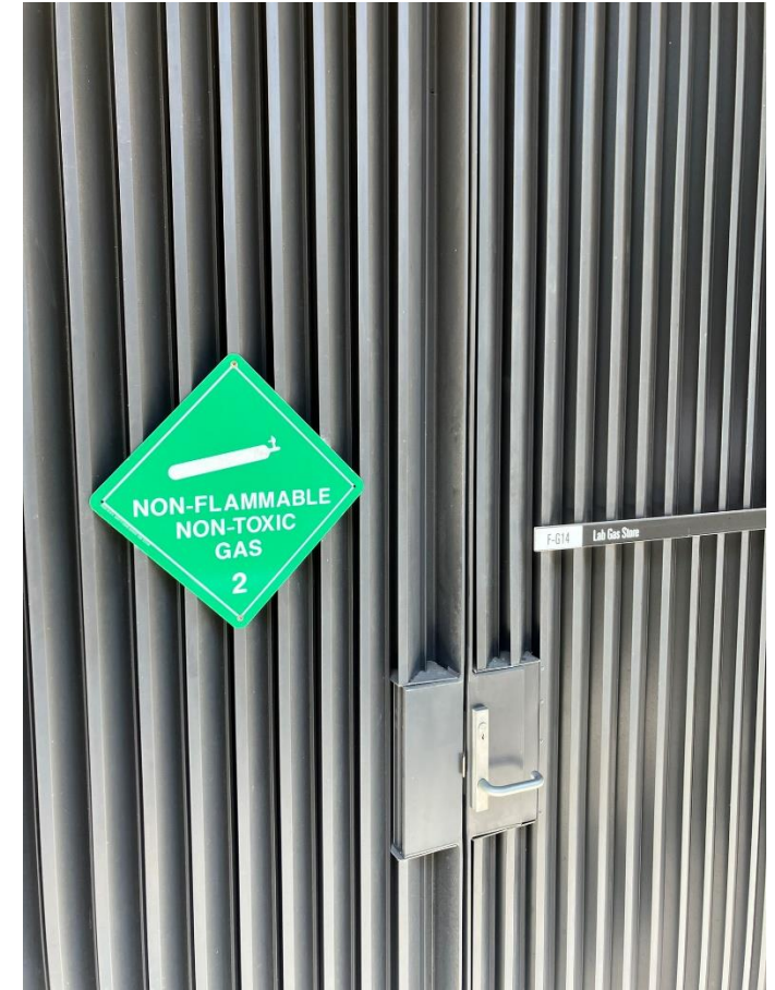
Figure 15 External Signage – Non-flammable Gas
