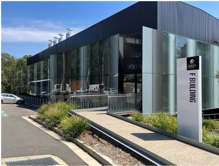
Figure 1 Entry to building kept clean and clear
