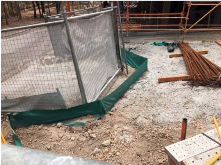
C29 – Evidence of Erosion & Sediment Control
