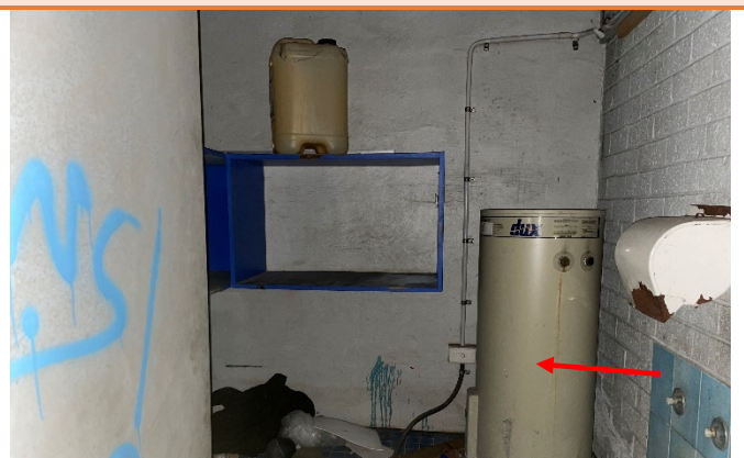
Photo 6 SMF in HWC ground floor store room
