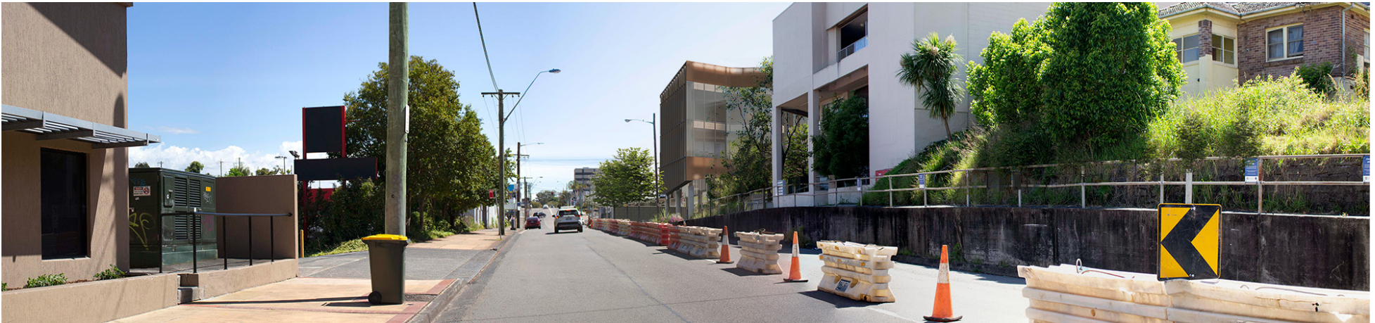
Image 42 Viewpoint 1, proposed view. Looking north from Mann Street outside Gosford Community Corrections Office. Indicative photomontage from this viewpoint of proposed works.
