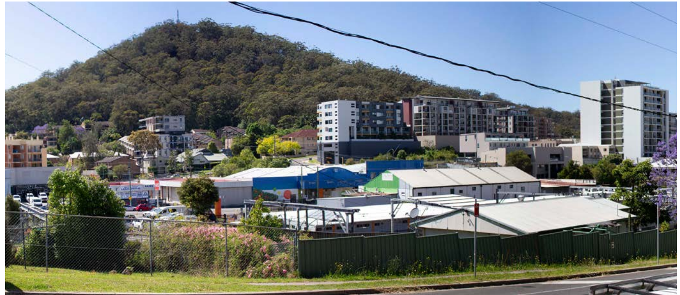
Image 55 Viewpoint 6, existing view. Looking south-east from pedestrian footpath/residential townhouse driveway at Etna Street/Showground Road roundabout
