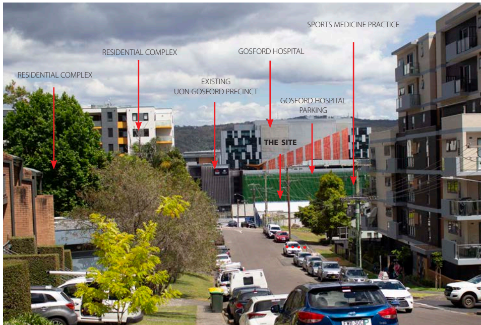
Image 2 Existing neighbouring sites, existing view looking west from Beane Street
