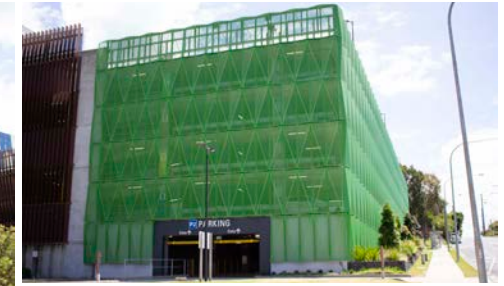
Image 29 Neighbouring Gosford Hospital parking along Showground Rd
