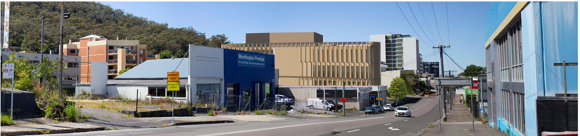
Image 54 Viewpoint 5, proposed view. Looking south-east from Etna Street/Mann Street roundabout. Photomontage from this viewpoint of proposed works
