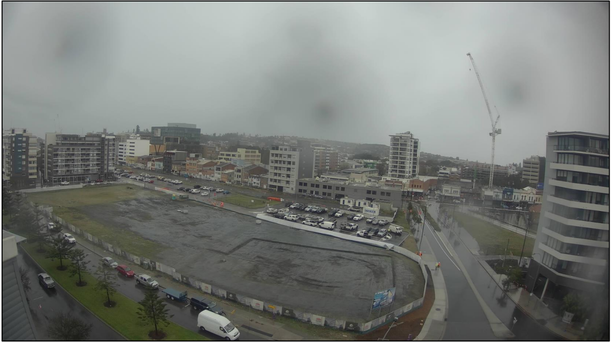
Figure 1: Photo of the site in the pre-construction condition.
